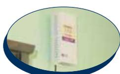
**Natural Gas Detector** - when the natural gas detector detects natural gas leaks, an alarm will be raised. It can also be linked to a complete gas shut off solution.
